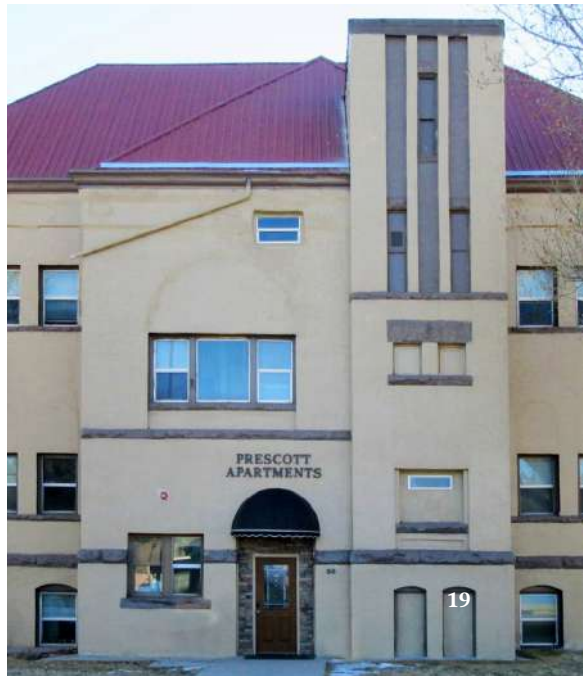
Eck House, 1217 West 4th Street (1917)
