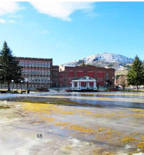
Waddell House, 506 West 3rd Street (1896) Washoe Brewery, 1200 East Park Avenue (1905) Glover Cabin, Washoe Park (1865) Anaconda Kennedy Commons, Band Shelter, Junior High School, and Daly Gym
