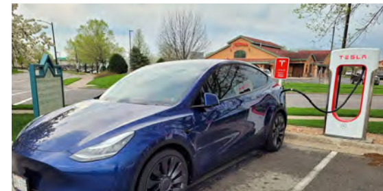
EV Charging Station - 2845 Midwest Dr
