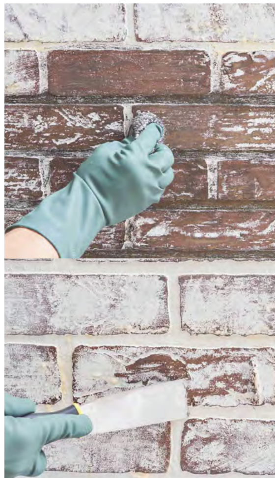
Clean and remove paint from masonry surfaces using gentle scraping methods.© The Spruce
