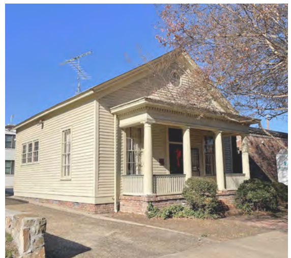
Preserve and maintain historic foundation materials that are in good condition. (610 S Rock St)
