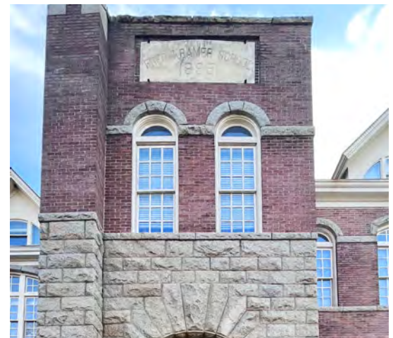
Upper story windows of Kramer School Lofts (715 Sherman St)
