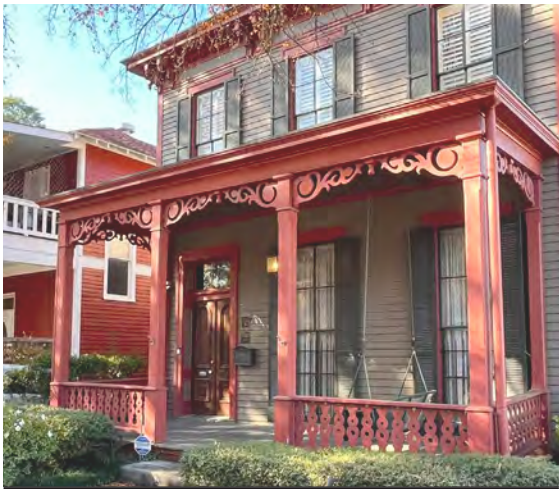
Maintain exterior painted surfaces through regular cleaning and repainting. (914 S Scott St.)
