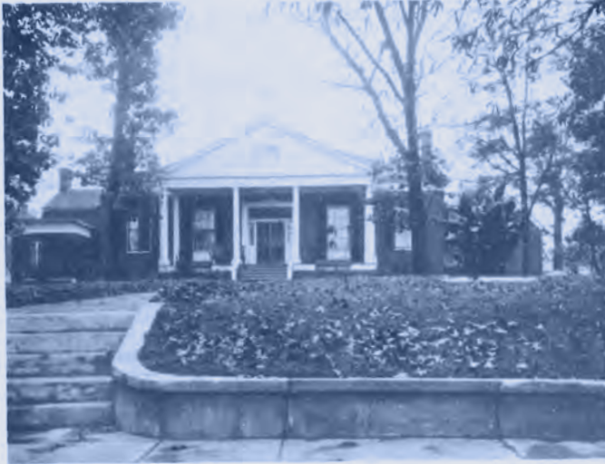
After Trapnall estate was settled in 1871, Trapnall Hall had several owners during the late nineteenth and early twentieth centuries. It was still a family residence when this photograph was taken circa 1910, but by the 1920s it had been turned into a boarding house. (Photograph courtesy of John Truemper.)
