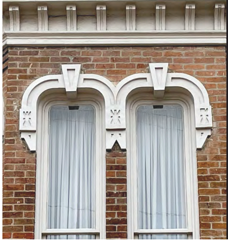
Lincoln House (301 E 7th St.)
