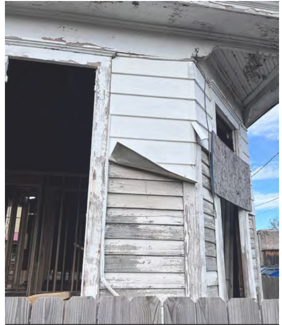
Remove existing artificial siding to uncover historic wood siding. (112 W. 13th St.)
