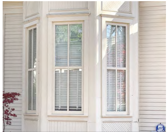
Maintain and repair window frames through repainting frames and replacing caulking. (609 S Rock St.)
