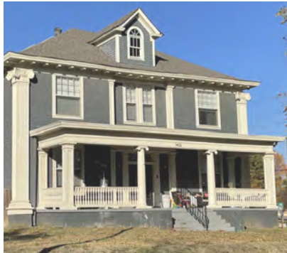
A Prominent dormer at Power House (1402 S. Commerce St.)
