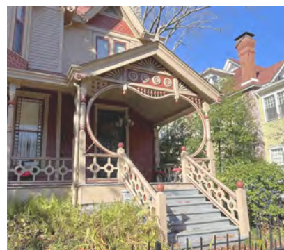
1010 S Scott St. retains its historic railing design.
