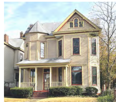
The porch at 915 Cumberland St has a shed roof.
