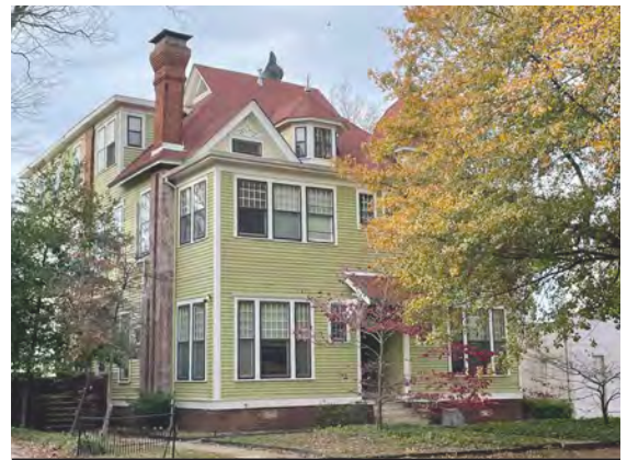
Retain and preserve original chimneys including brick pattern, shape, and color. (Ratcliffe House at 1004 S. Scott St.)
