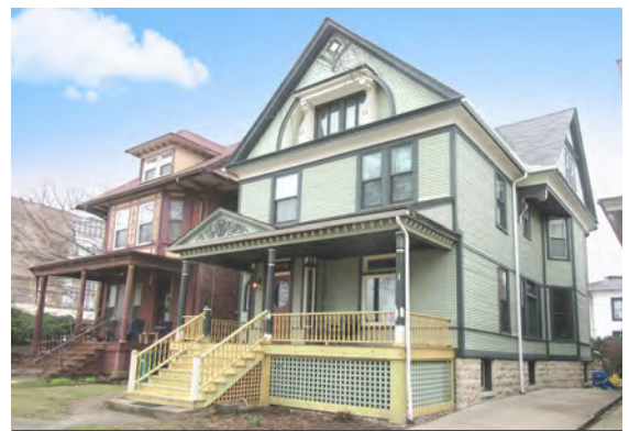
Replace deteriorated historic porches, if necessary, using in-kind materials matching detail, size, and profile. @ Village of Oak Park, IL
