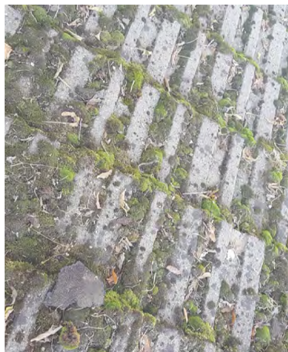
Look for patches of moss or biological growth when inspecting a roof. © Village of Oak Park, IL
