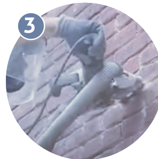
MORTAR SAWING
