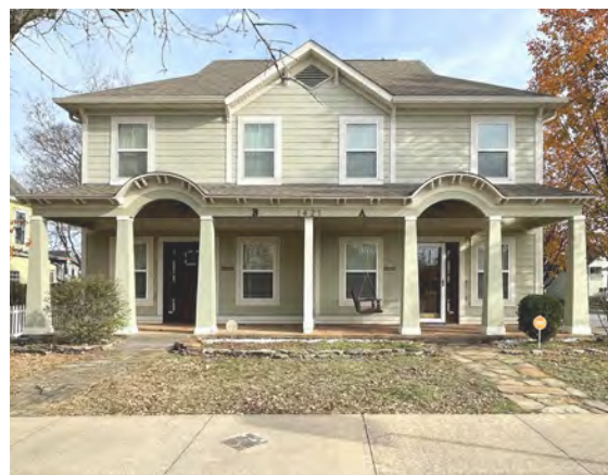
New roof areas should be compatible with the roof forms, types, shapes, and pitches found within the area of influence. (1421 Cumberland St.)
