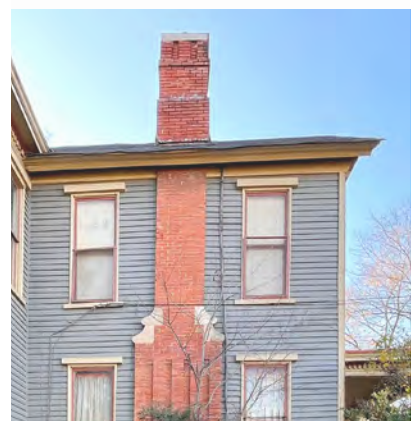
The Litzke House 521 E 8th St. features several elaborate chimneys.
