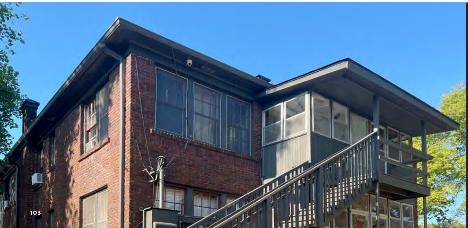
Place new staircases and fire escapes in areas minimally visible from the public right-of-way. (524 E. 6th St.)
