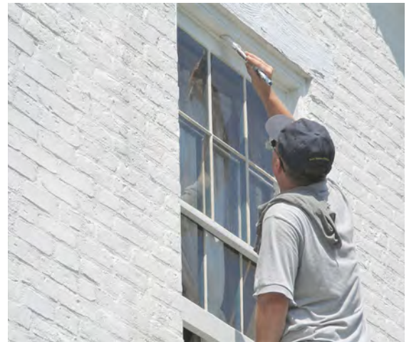
Scrape and repaint historic windows to protect wood from deterioration. | © Indiana Landmarks
