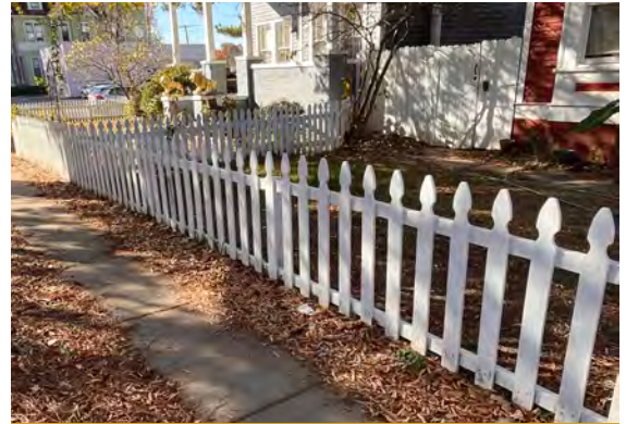
Retain and preserve front yard fences. (916 Scott St.)
