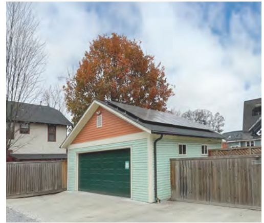
A side gable garage roof with solar panels. (1410 S. Rock St.)
